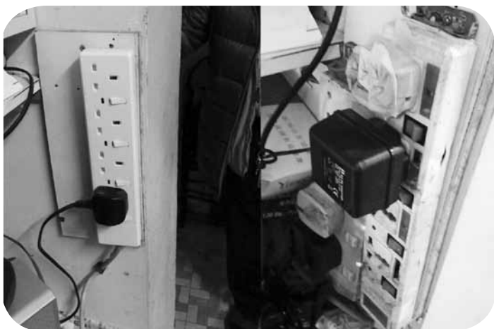
圖右為不正規拖板，圖左為更換後的正規拖板。 Standard multi-socket extension lead on the left replaces that on the right which is not in standard.
