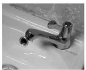
更換手撥式水龍頭,減少長者囤積食水 情況,去除地面濕滑而跌倒的危機。 Replacement by lever type faucet reduces spilling of bucket water and hence eliminates risk of fall due to wet flooring.
