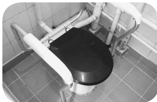
廁板扶手的設計與一般的扶手完全不同，兩邊的扶手延伸到地下，使體弱長者能更安心用力協助站立。 Toilet Safety Frames serve functions different from grab handrail: The grab handrails on both sides extend to the floor and help elderly stand on a secure footing.
